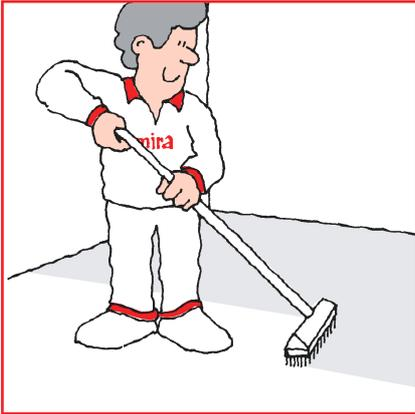
Prime all cement based surfaces with 1 coat of 4120 sealer diluted with water, 1:3. Do not prime plywood surfaces.
