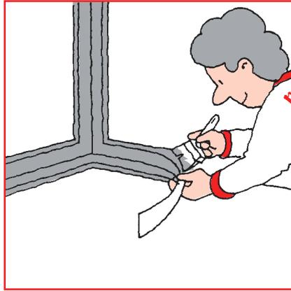
Cover all joints, edges and corners with 100 mm wide safecoat strip pressed into a coat of 4400 multicoat. Screws in plasterboard should also be covered with 4400 multicoat.
