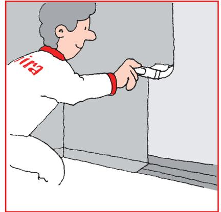
In the "damp-zone" (see diagram on back page) a min 100 g/m<sup>2</sup> of 4120 sealer should be applied.
