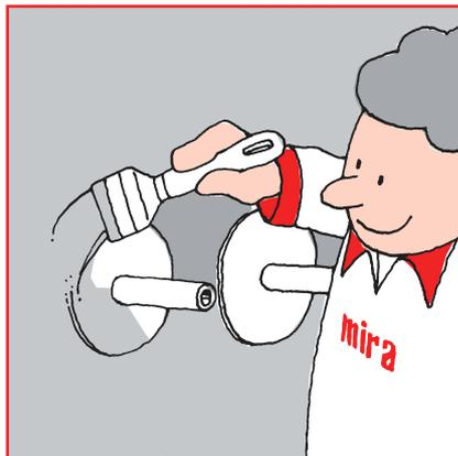
After fitting the safecoat manchete, firmly spread 4400 multicoat so that it is fully covered and the material is saturated.
