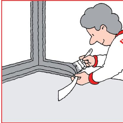
At the floor/wall joint use the 100 mm safecoat strip pressed into a covering of 4400 multicoat.
